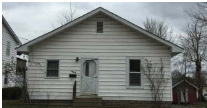
1105 WHITE, MARION. House being sold AS IS. Owner is long-time owner, but hasn't lived there for years. Tax records count the enclosed back porch, but that's not real living space. Also, tax records list 1935+/- as the age. Owner thinks it might be closer to 1925.
