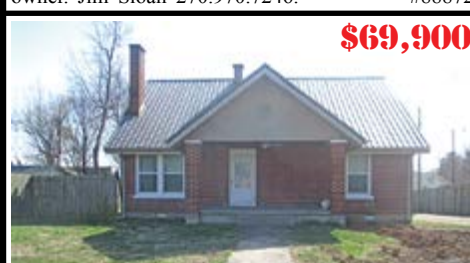
$69,900 1336 W BROADWAY ST. - Charming Brick homew ith 2 bedrooms and 1 bath home with beautiful hardwood floors and with many updates. Metal roof, windows, insulation, heating & air, and plumbing all done 10 years ago. All kitchen appliances stay plus washer & dryer. Large lot with 1-car garage & carport and outbuilding. $69,900. Call Mary Ann 270-705-1132. #89563
