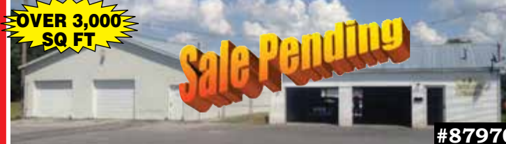
OVER 3,000 SQ FT Sale Pending #87970 355 & 375 BIRCH ST, BENTON, KY - 2 Commercial Buildings in Benton. Perfect for Auto Clean-Up, Body Shop, Storage, etc. Use one building and rent the other to pay the bills!! Unlimited possibilities! $89,900
