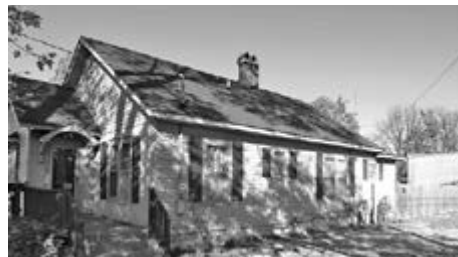
206 N Jefferson St. W.F. - 3 bedroom. Office could be used as 4th bedroom. Both bathrooms are remodeled. Very big living room. Small basement for safety & storage. The Privacy Fence hides the great layout of the backyard. Detached garage. New furnace unit 6/2016.
